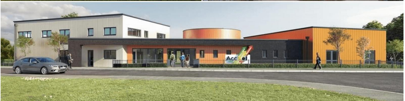
AccXel – Construction Skills Centre, Cinderford - For more details see: www.accxel.co.uk
