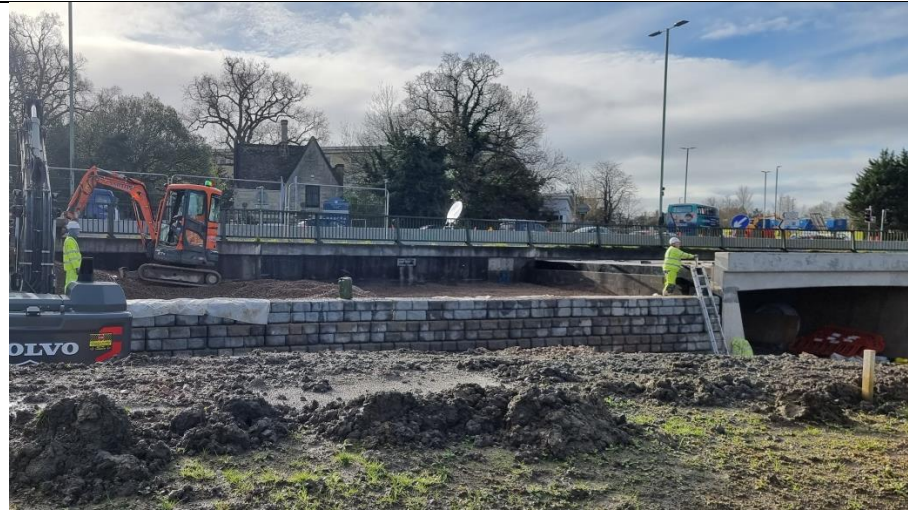
Photograph 4: Subway Retaining Wall Construction
