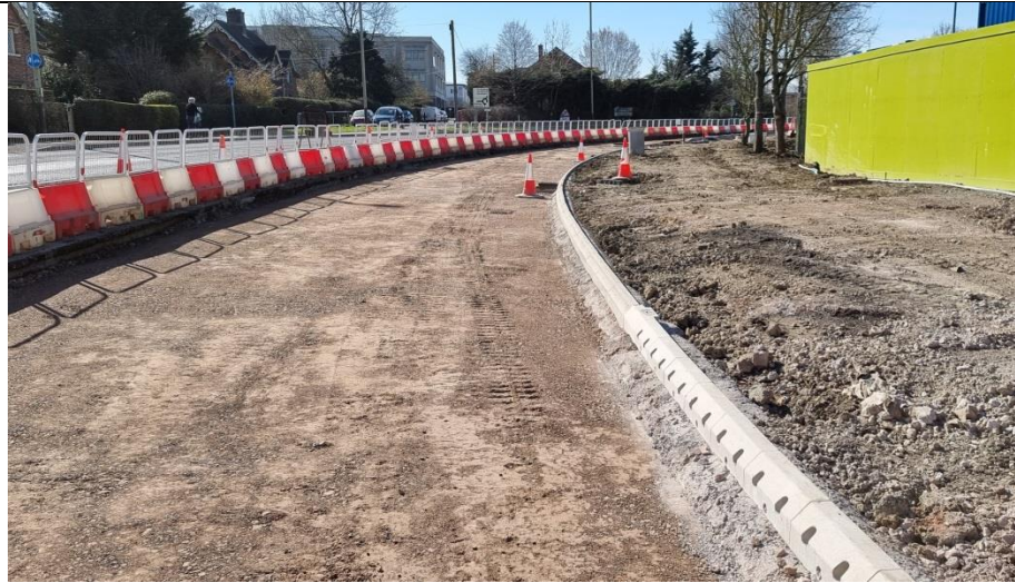
Photograph 2: Widening of Carriageway on Hatherley Lane
