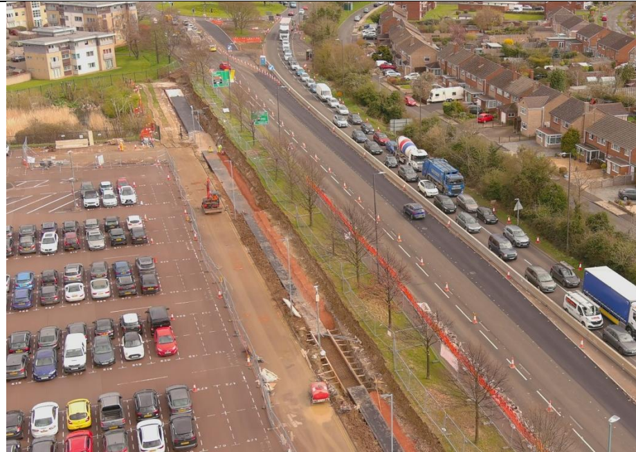
Photograph 5: Construction of GCHQ Retaining Wall
