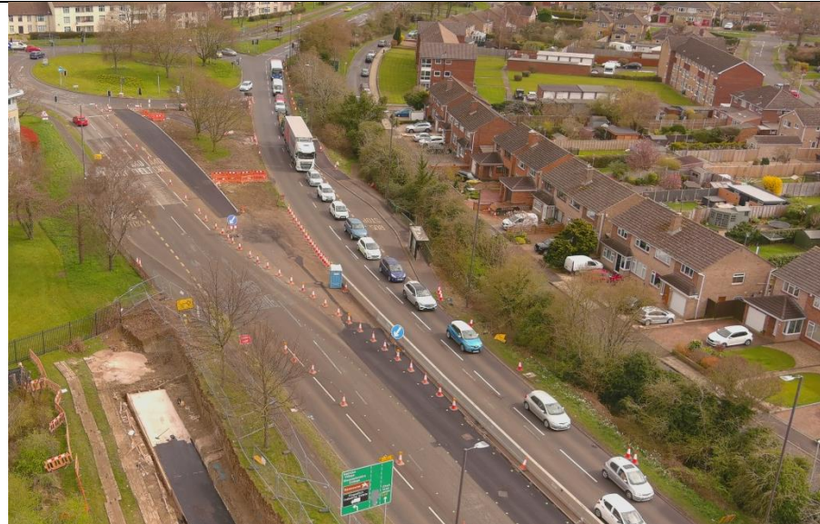
Photograph 7: A40 Eastbound Carriageway Widening approaching Benhall Roundabout
