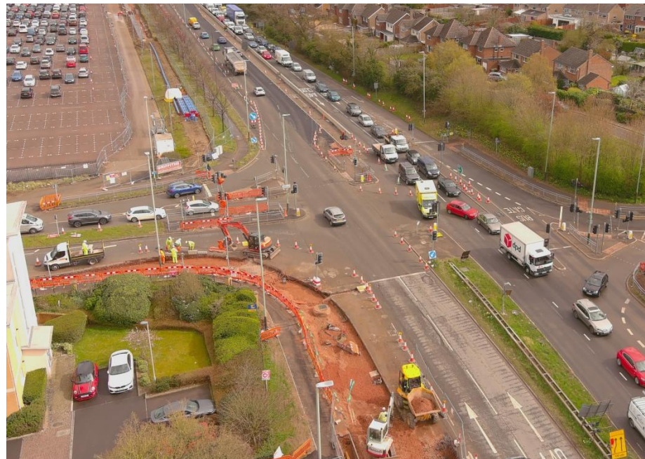
Photograph 6: Telstar Way Junction Widening Works
