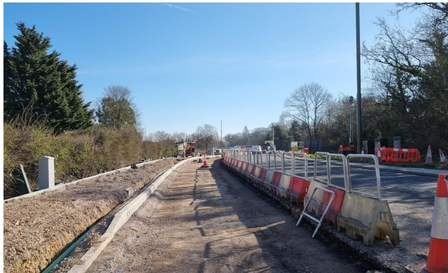
Photograph 3: Widening on the B4063 for New Bus Lane
