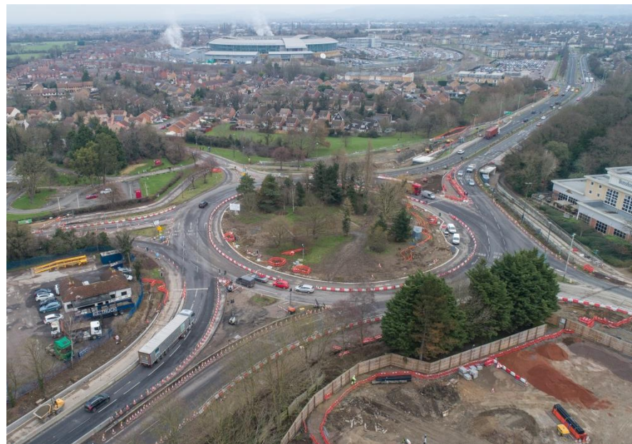
Photograph 1: Widening Works on Arle Court and approaches (January 2021)
